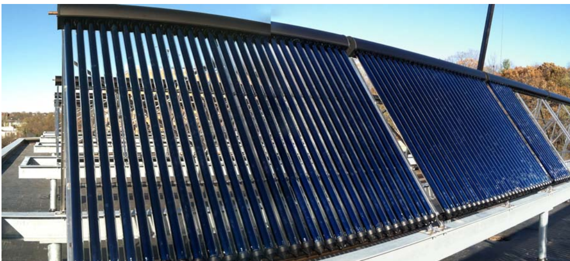
Installation of solar hot water at Park Tower Apartments
