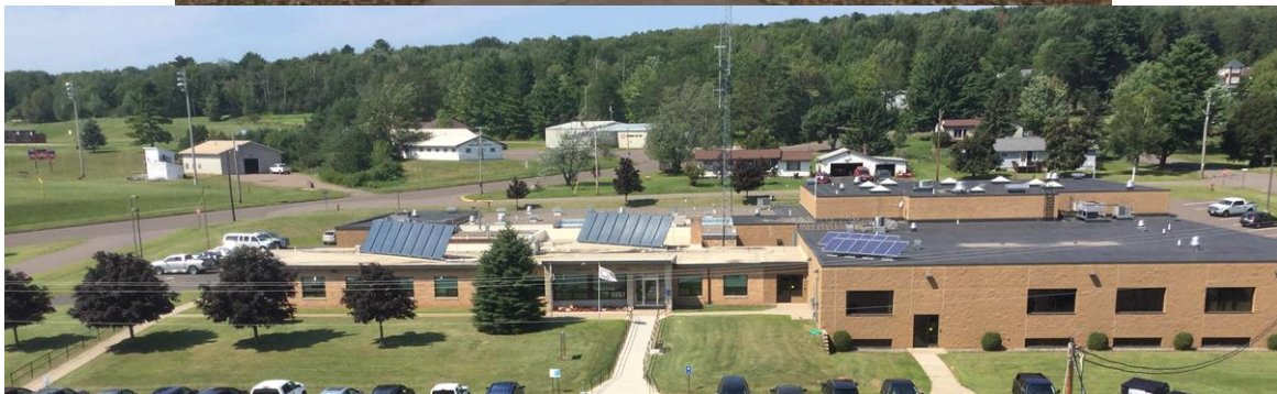
Bayfield County Courthouse and Solar Thermal and Solar PV panels on the Annex and Jail.
