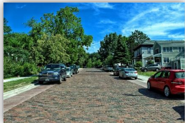
North Broad Street postconstruction.
