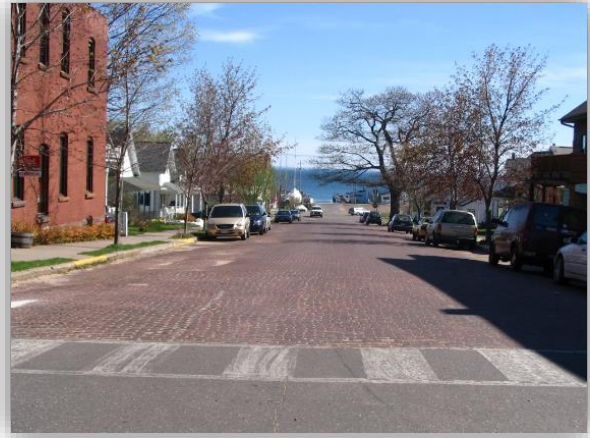
Before construction: South Second Street.
