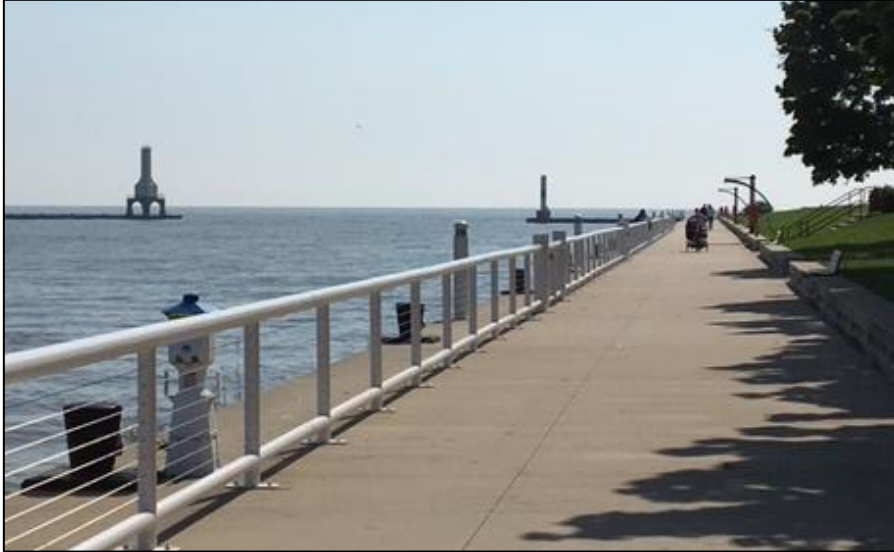
Coal Dock Park water's edge railing (City of Port Washington)
