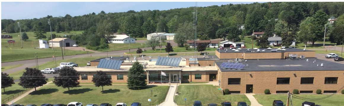
Bayfield County Courthouse and Solar Thermal and Solar PV panels on the Annex and Jail.
