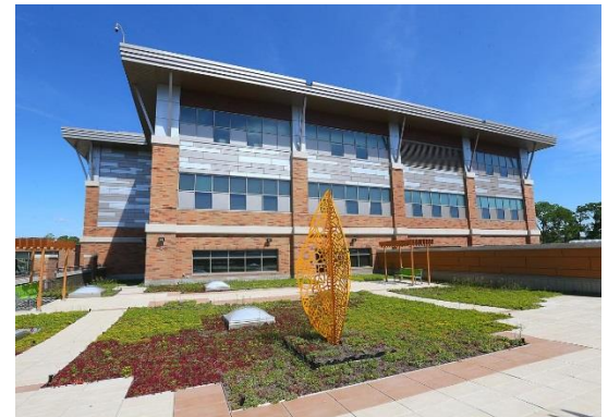
Western Technical College Integrated Technology Center. Source, La Crosse Tribune
